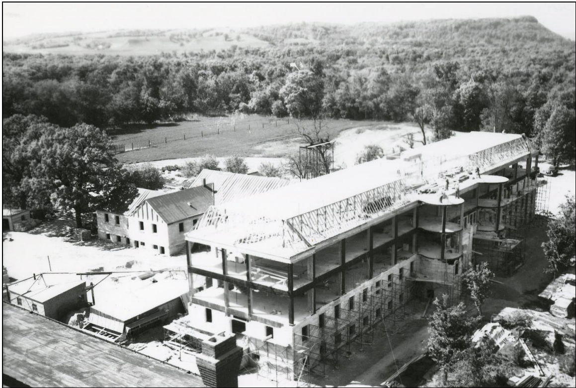
Marian Hall construction, 1945
